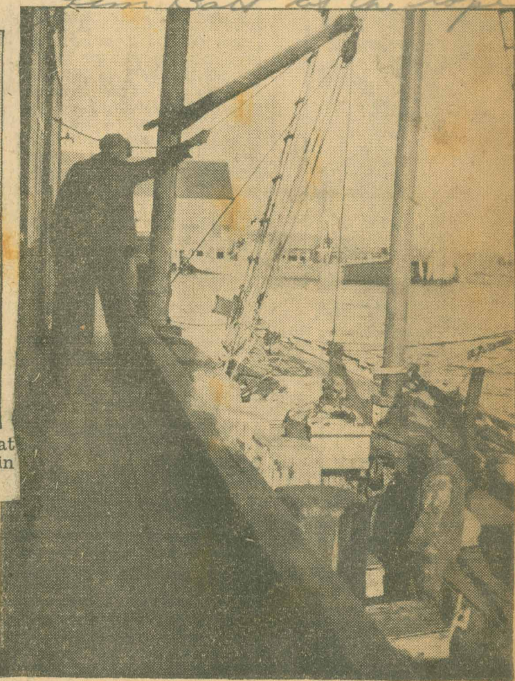
The steam winch at Sklaroff's wharf, Provincetown, brings up a box of fish from the deck of the Barbara C.
