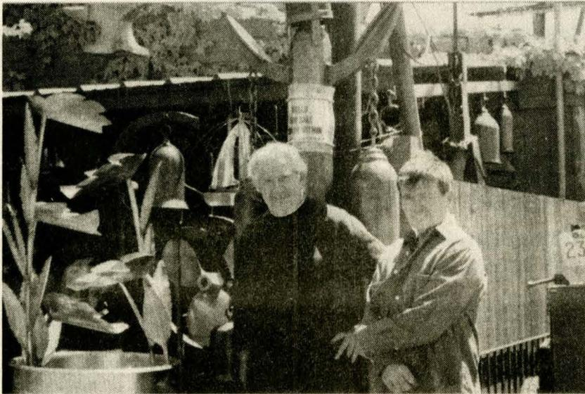
Bells made from recycled helium, CO2 and scuba tanks—their "Bells by the Pound"—are a constant and steady shop turn-out. Clarence and son Michael extend the life of these rejects by cutting the top down to the desired length and then forming the bell shape by lowering a forge-heated and glowing cylinder. This spreads the opening to a flared rim. After the cylinder has been
