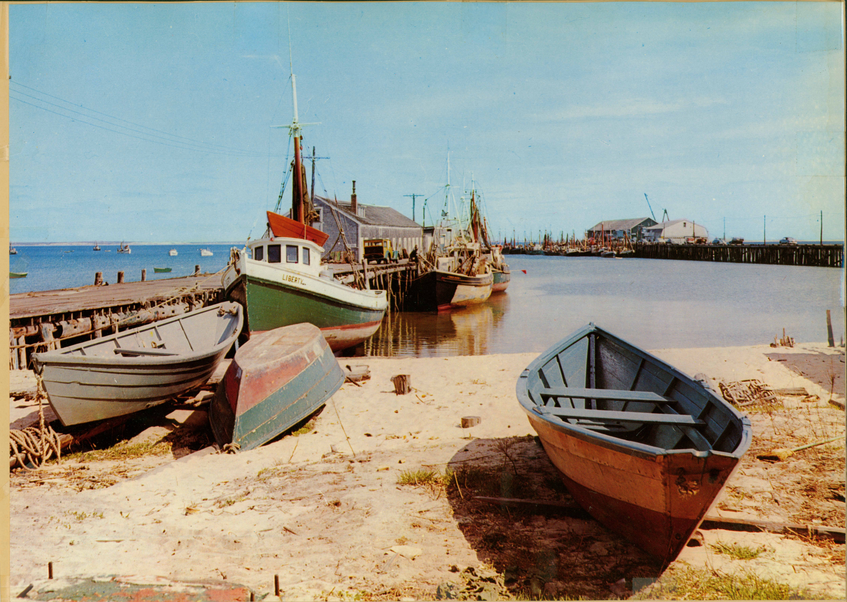
A 1955 view of the J.D.Hilliard Wharf, left (and Railroad Wharf, right,) with Higgins Lumber shed on the end of Hilliard's
