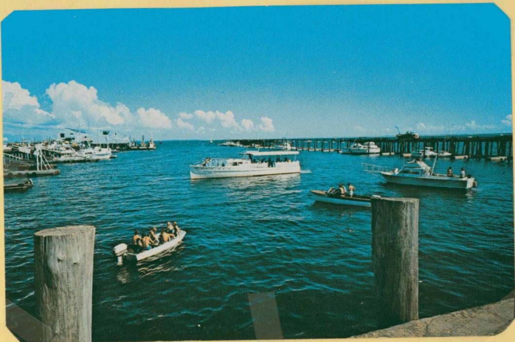
Railroad, or MacMillan Wharf, left, and the now repaired Fisherman's Wharf, right 1980
