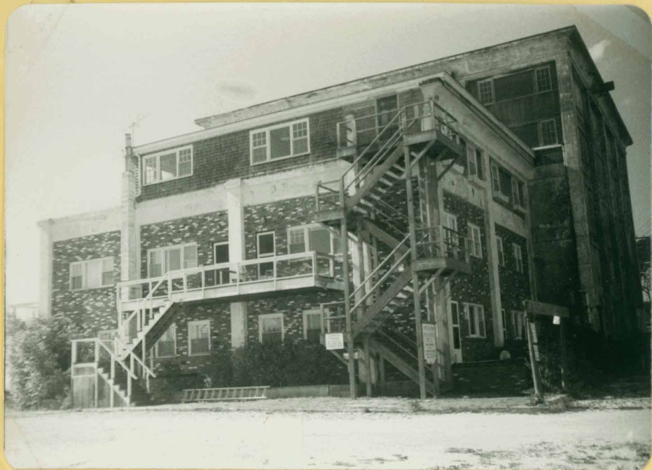
Consolidated Cold Storage opposite Hancock Street, now made into apartments - October 1980
