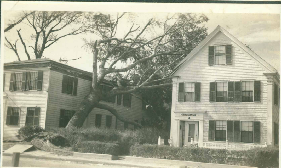
Near Ark. Assoc. Building Sept. 14. 1944
