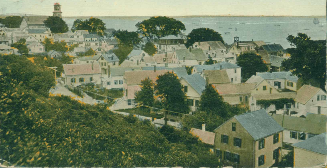
View from Town Hall looking East, Provincetown, Mass.
