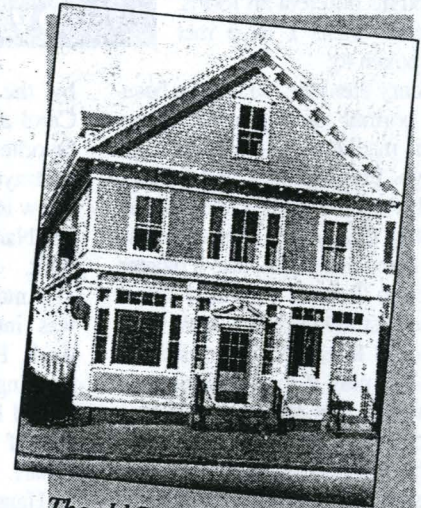
The old Seamen's Savings Bank building
