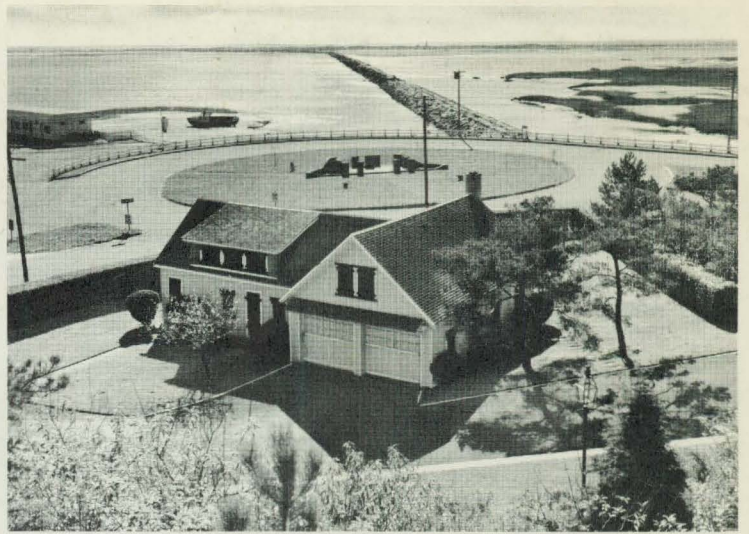
View over Gate House from Residence
