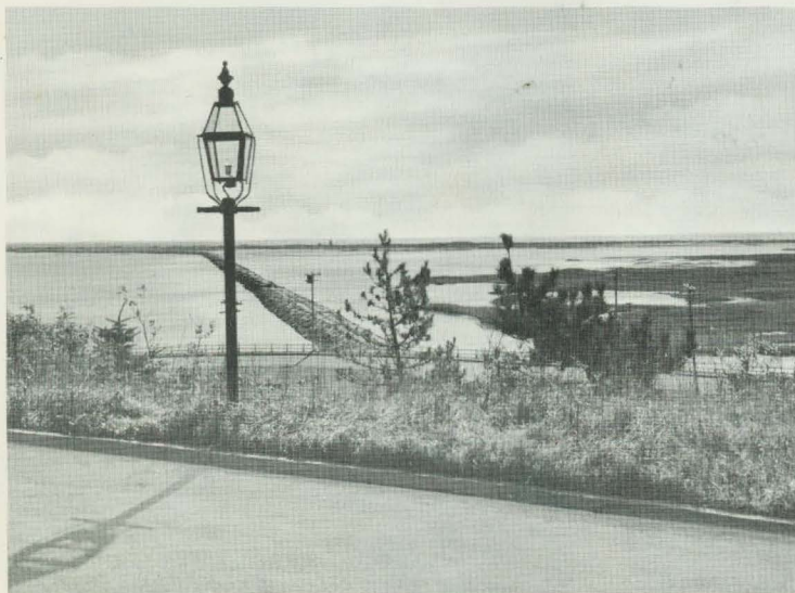
View from Lower Driveway
