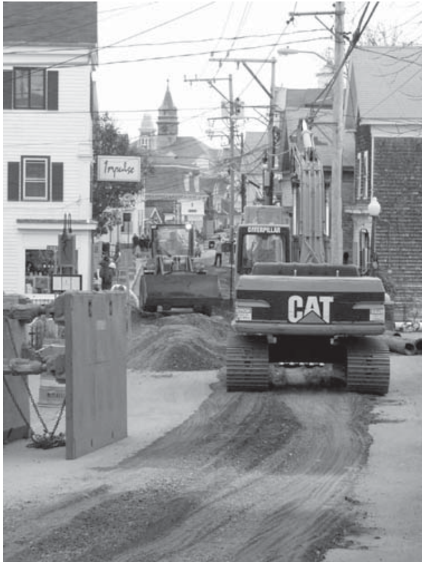
Sewer construction along Commercial Street - 2003.
