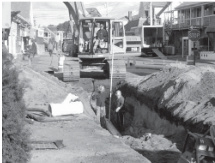
Sewer construction on Bradford Street (top) and the corner of Standish and Commercial Streets (below). Over 650,000 feet of sewer pipe was installed throughout the town in 2003.
