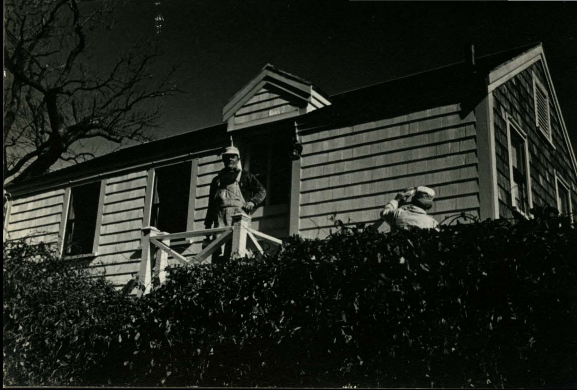
40 Commercial Street - rear apartment circa 1945-6 - getting a fresh coat of paint
