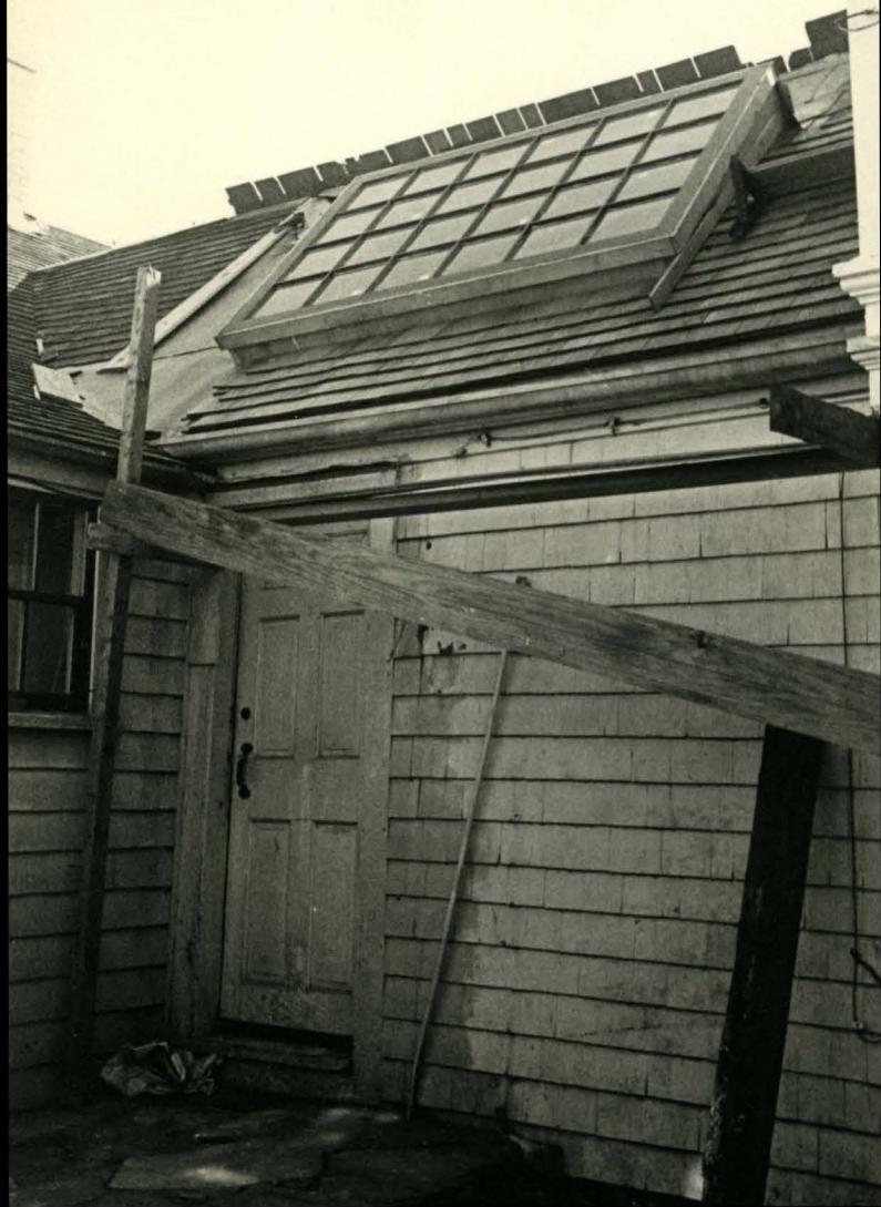
40 Commercial Street circa 1945-6 - undergoing renovations Installation of multi-paned skylight
