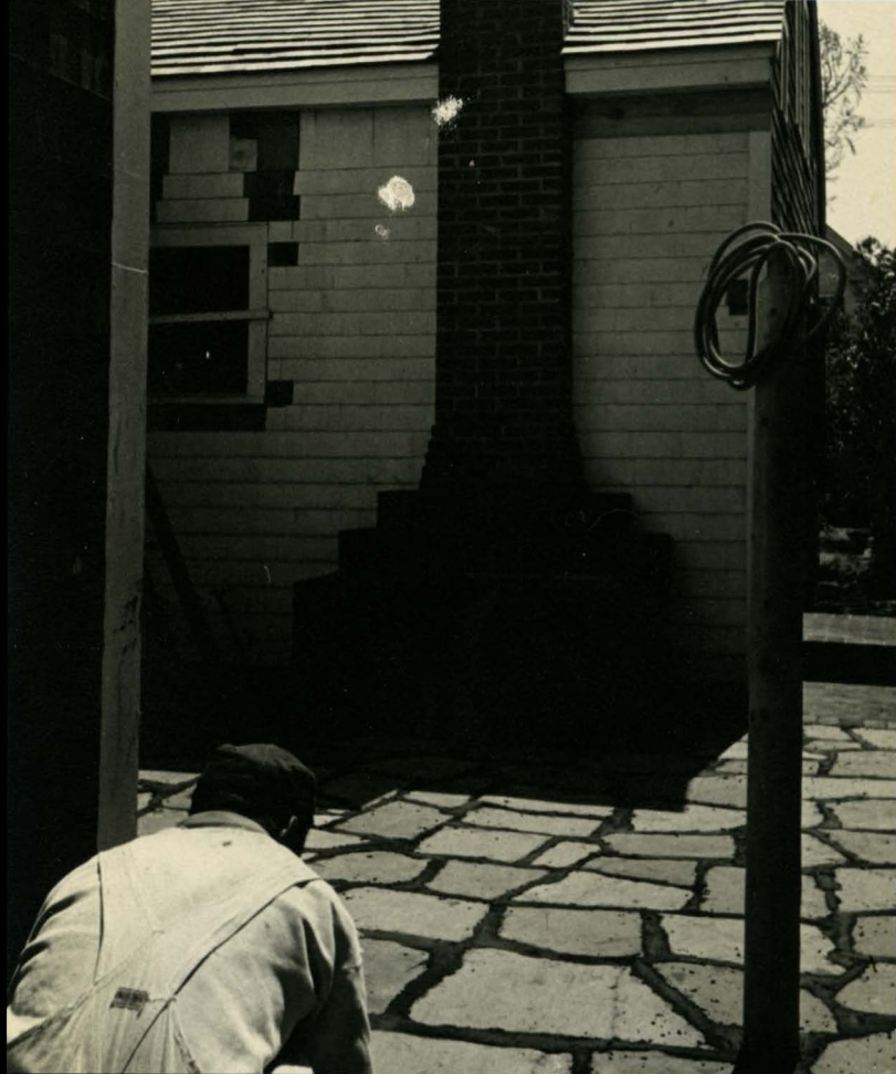
40 Commercial Street - circa 1945-6 Patio flagstone being laid
