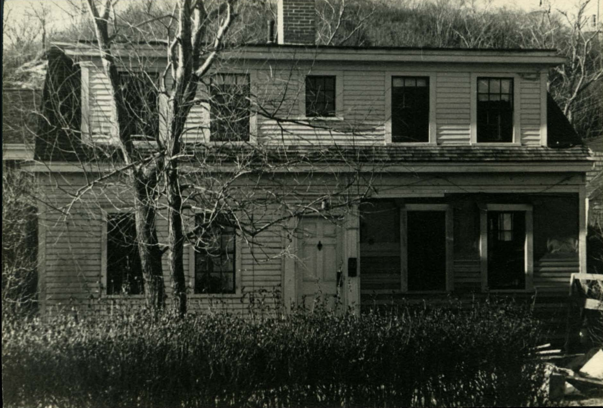
40 Commercial Street circa 1945-6 Undergoing renovations
