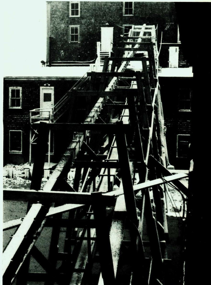
Aerial cableway at the Cape Cod that took the fish from the trap boats to the packing section on the fourth floor.
