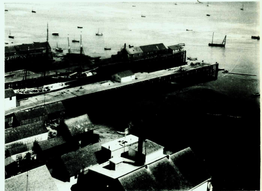
The Provincetown (along the lower edge of the photo) as seen just after it was built about 1895. Note aerial cableway with fish carrying box suspended from it.
