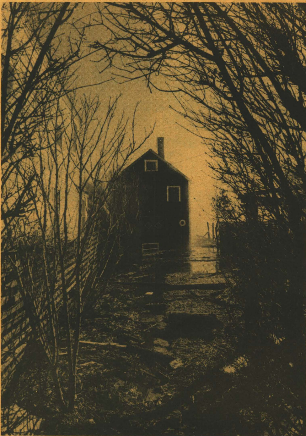
West End lane after flood (see photo bottom right). Advocate photo by Gregory Katz
