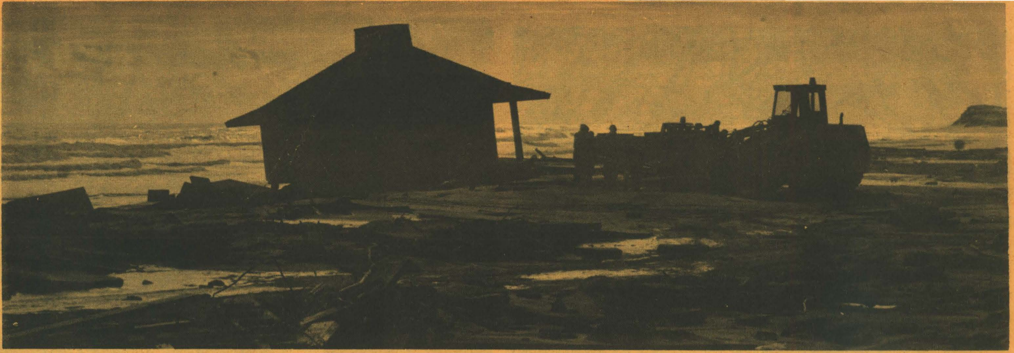
Coast Guard Beach bathhouse had to be destroyed by fire before it washed out to sea.
