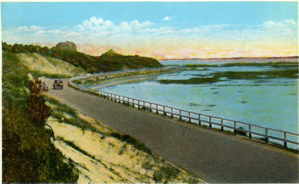
148 DRIVE ALONG THE NEW STATE ROAD, PROVINCETOWN, CAPE COD, MASS.
