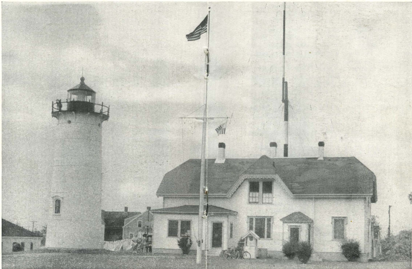
CHATHAM LIGHTHOUSE AND U. S. COAST GUARD STATION
