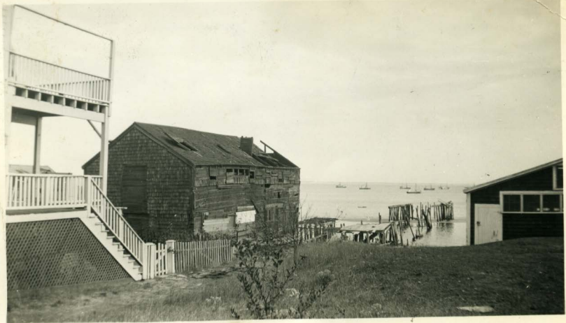
Remains of Old Canning Factory & Wharf. Opposite Law Street After Hurricane.
