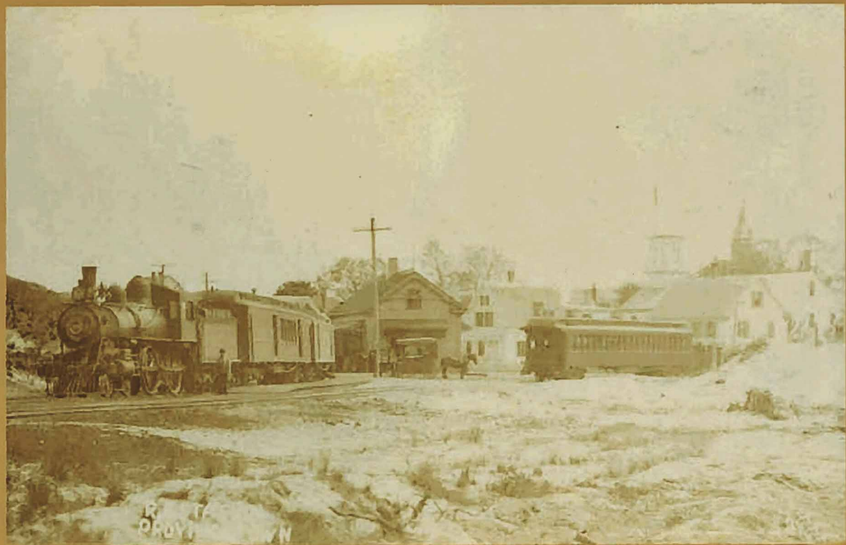
The Railroad Station from the Rear. - 1880 Center School & Town Hall on right.
