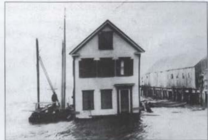
One of the fishermen's houses being moved by boat from Long Point to the mainland when the community shifted away from the point.
