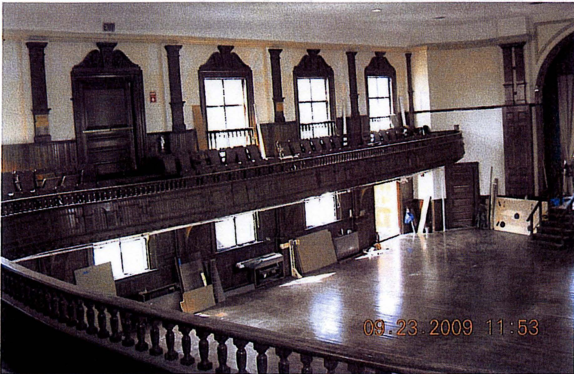
Figure 4. Present appearance of South wall or balcony.
