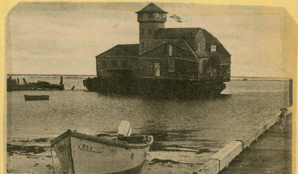
Barge carrying lifesaving station floats parallel to beach after a mooring line to Macara's Wharf snapped. Station was moored alongside wharf.
