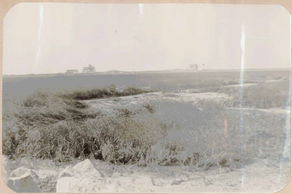
The Station and Light from the Breakwater -- Sept. 1944
