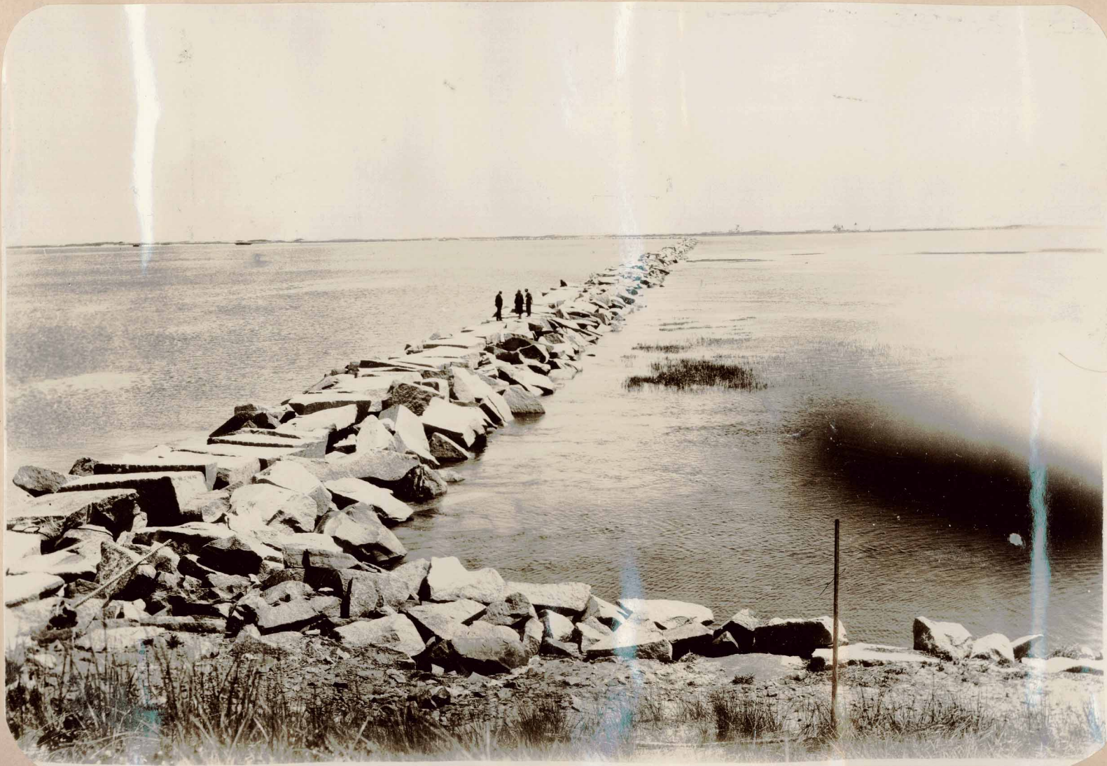
..... A John R. Smith photo of the new breakwater.
