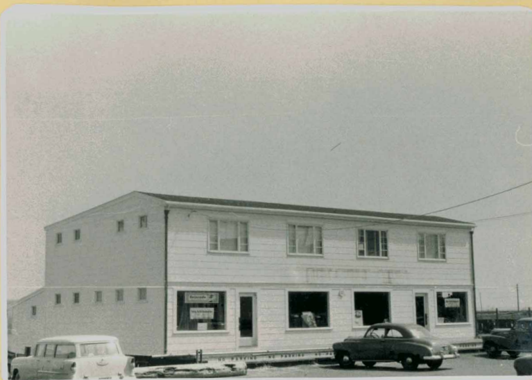
Land's End Marine Store (behind the main store, and where McGuire's Sail-loft used to be. June 1, 1956
