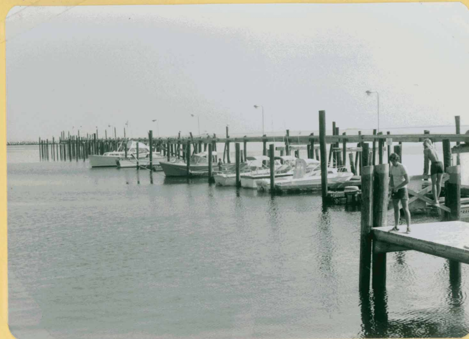
New Boat Slip where Sklaroff's Wharf was - Sept. 1977 -
