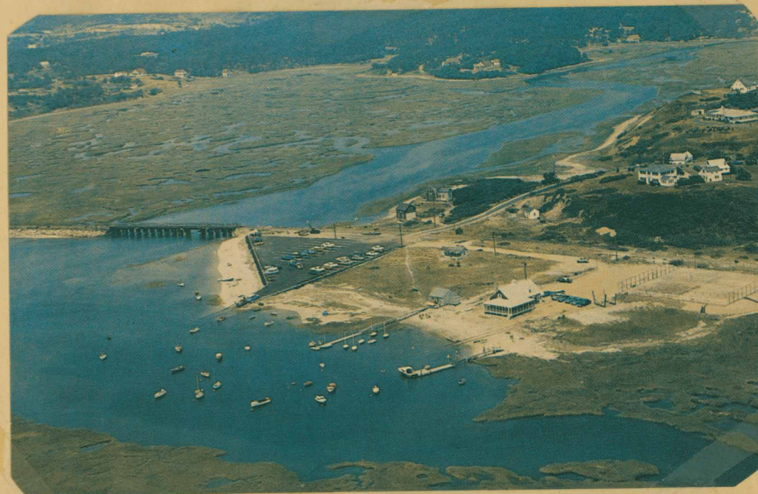
Air View - 1960 - Showing Pamet River Bridge
