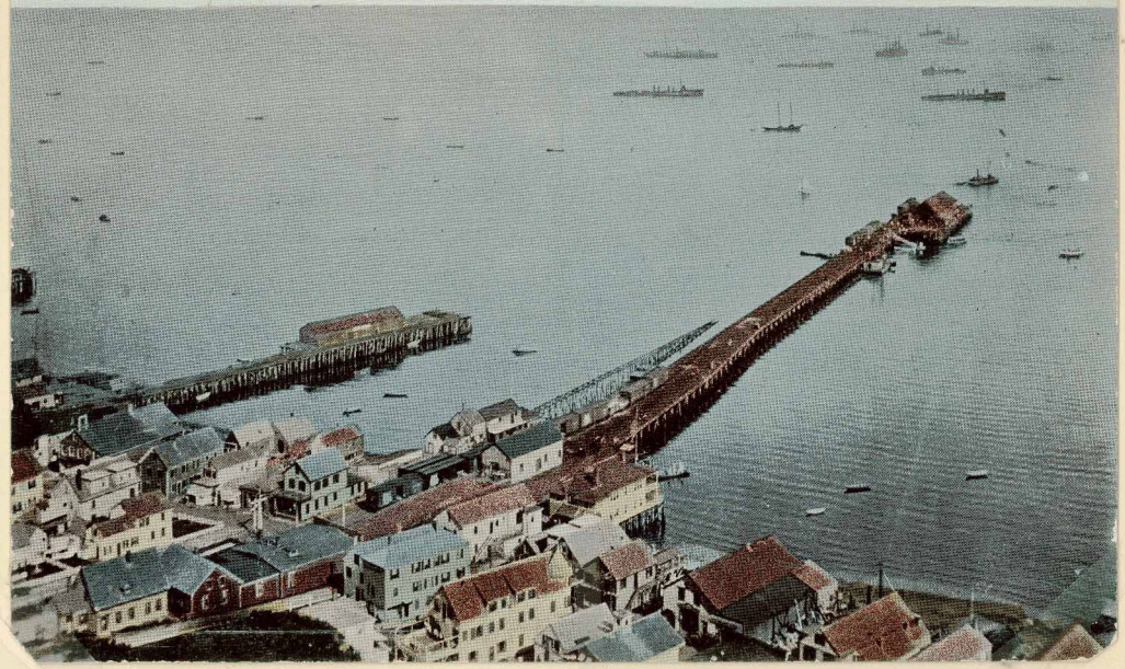
Hilliard's Wharf left, Town Wharf, Right - 1909
