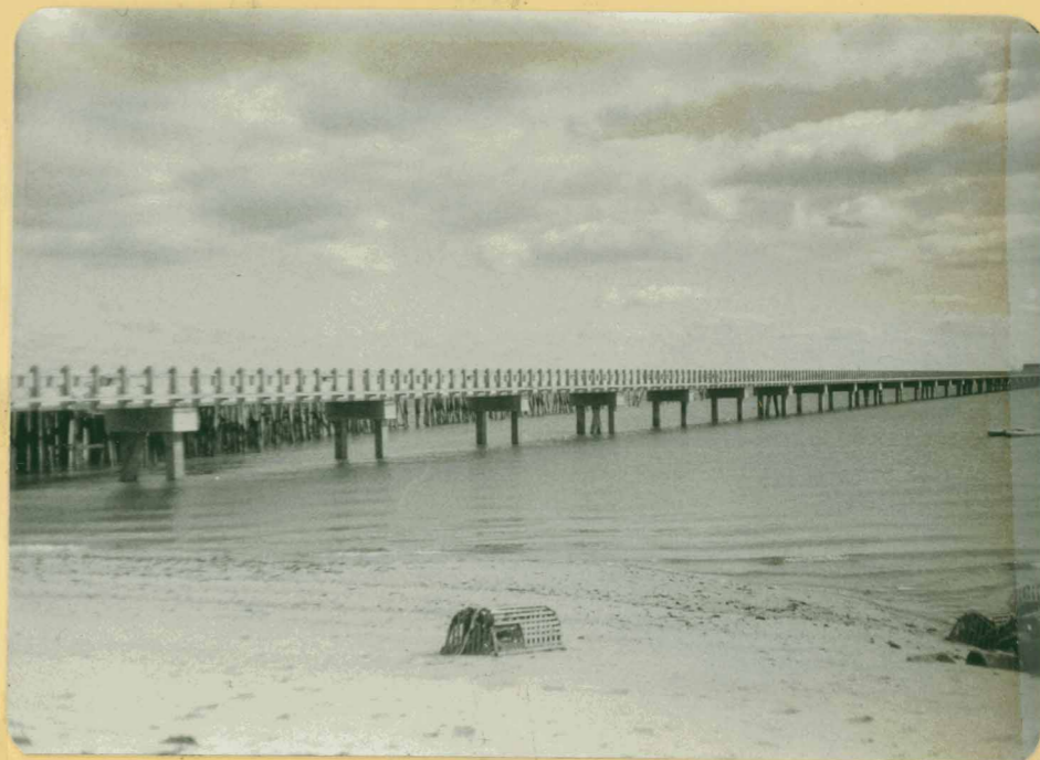
New Coast Guard Pier with the old Freeman Wharf underneath - Oct. 1980
