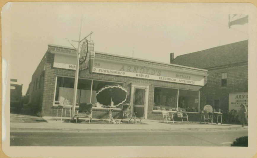
The new store finished. Taken Sept. 1952
