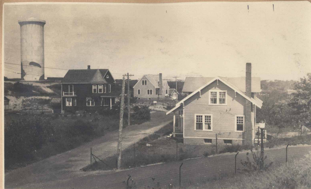
Same view about 1940 with John R's house, right. Note new standpipe. Road to Monument, right.
