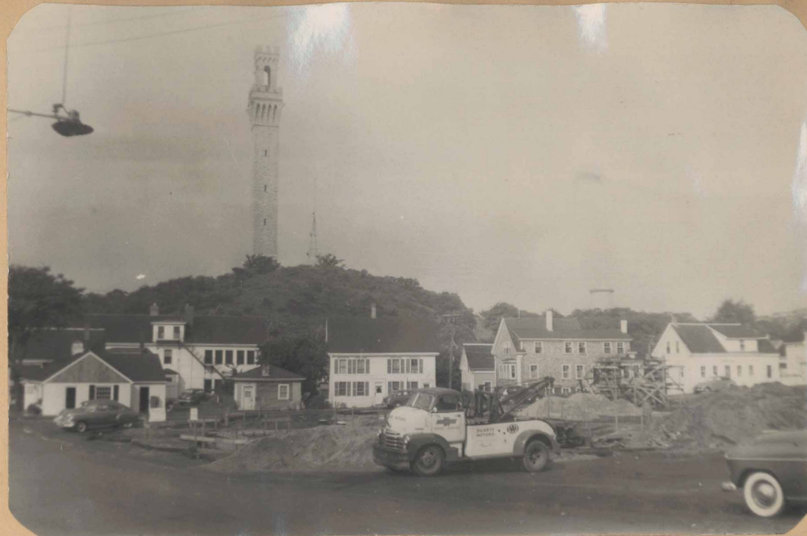
Breaking ground for new garage.
