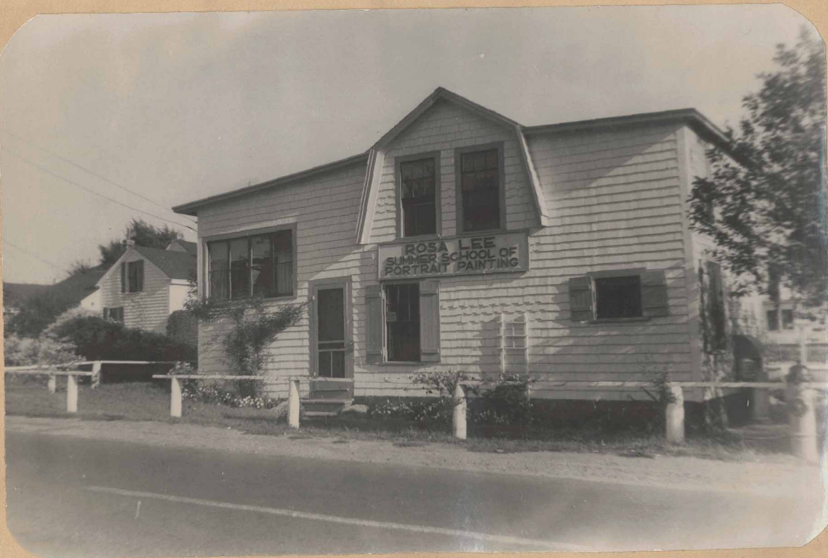
Bradford St. corner Kendall Lane (left) and opposite the Atkins Mayo Road - Sept. 1951
