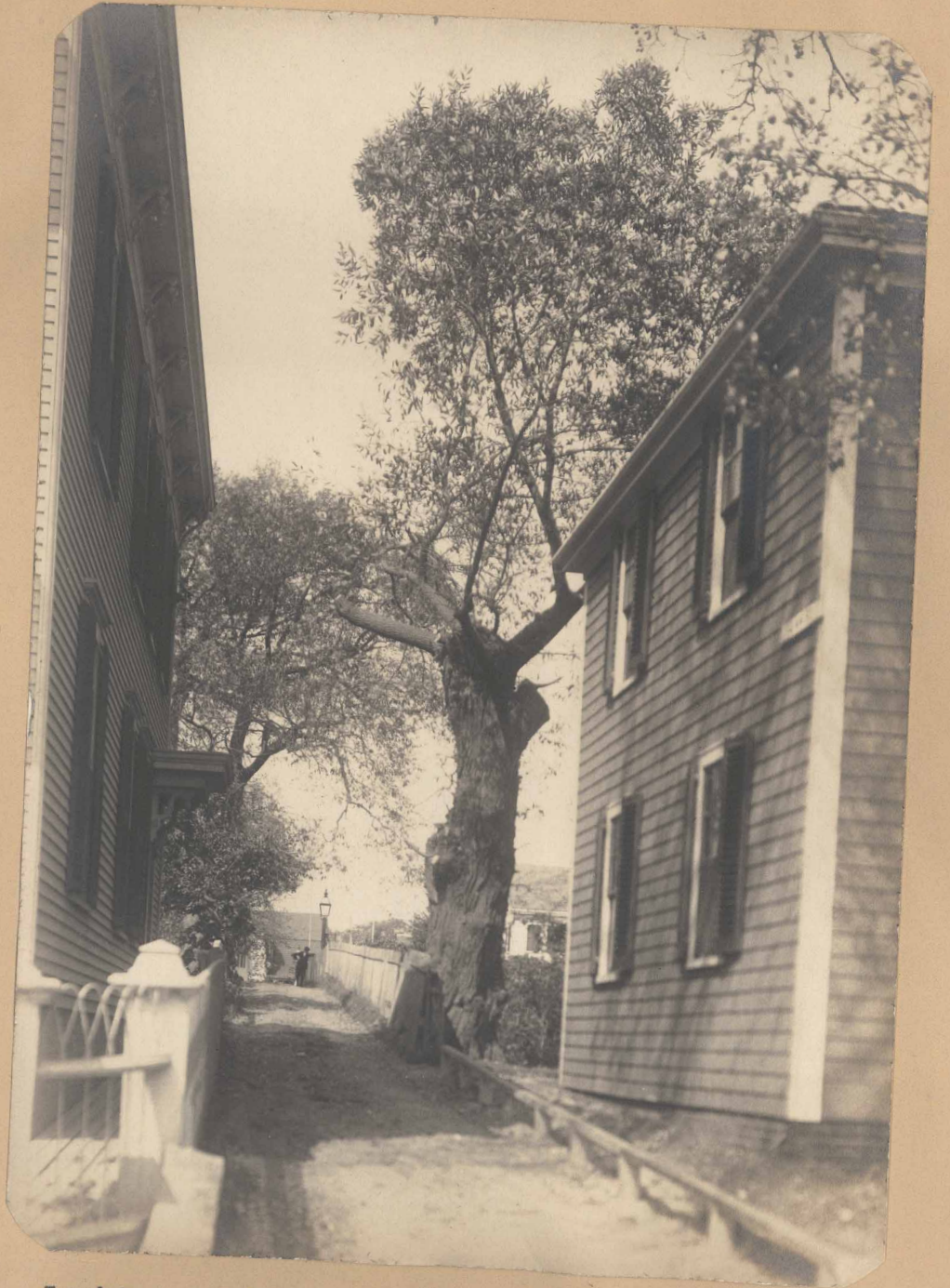
Looking up Law Street from Commercial - 1910 (Opposite Pickett's Canning Factory)
