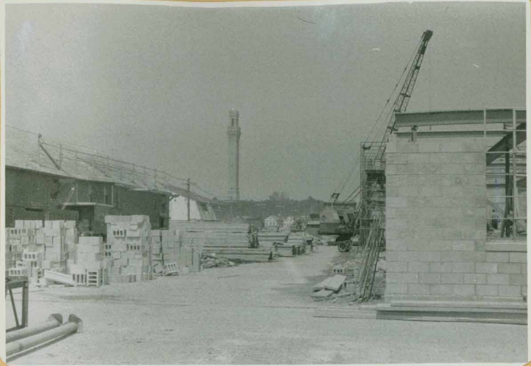
Old Wharf, left; new one, right. June 1956
