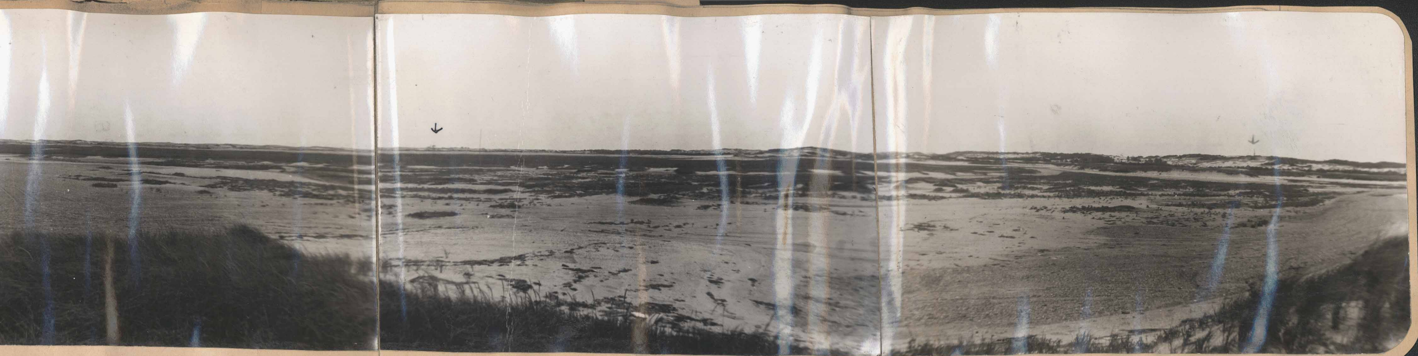
left. Arrow: Steam Shovels and trucks working on the dike. Pilgrim Monument may be seen on the far right.
