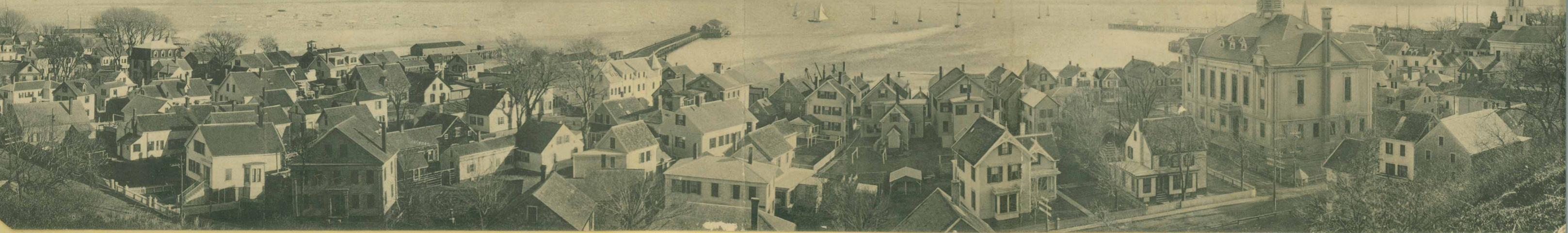
Another of the Harbor from Town Hill - About 1910 - Library, left under big tree. Cupola: Used to be 1st schoolhouse on Long Point. Railroad Wharf, with Steamboat Wharf (from Court Street) on the right. Christopher Wren Church, right.
