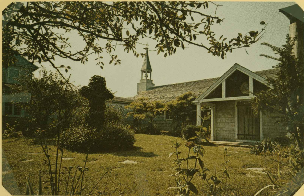
Side view showing the S-4 Cross (See story ahead on this submarine disaster) - 1964
