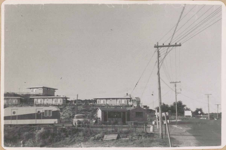
Here are our new type "Motels" Corner of West Vine and Bradford Streets. Facing West - September 1953
