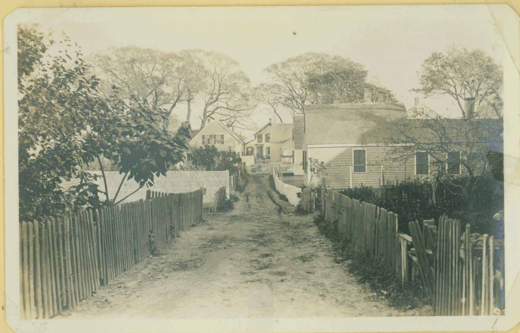
Down West Street from Bradford - 1945 - This Street is next street West to Soper St.
