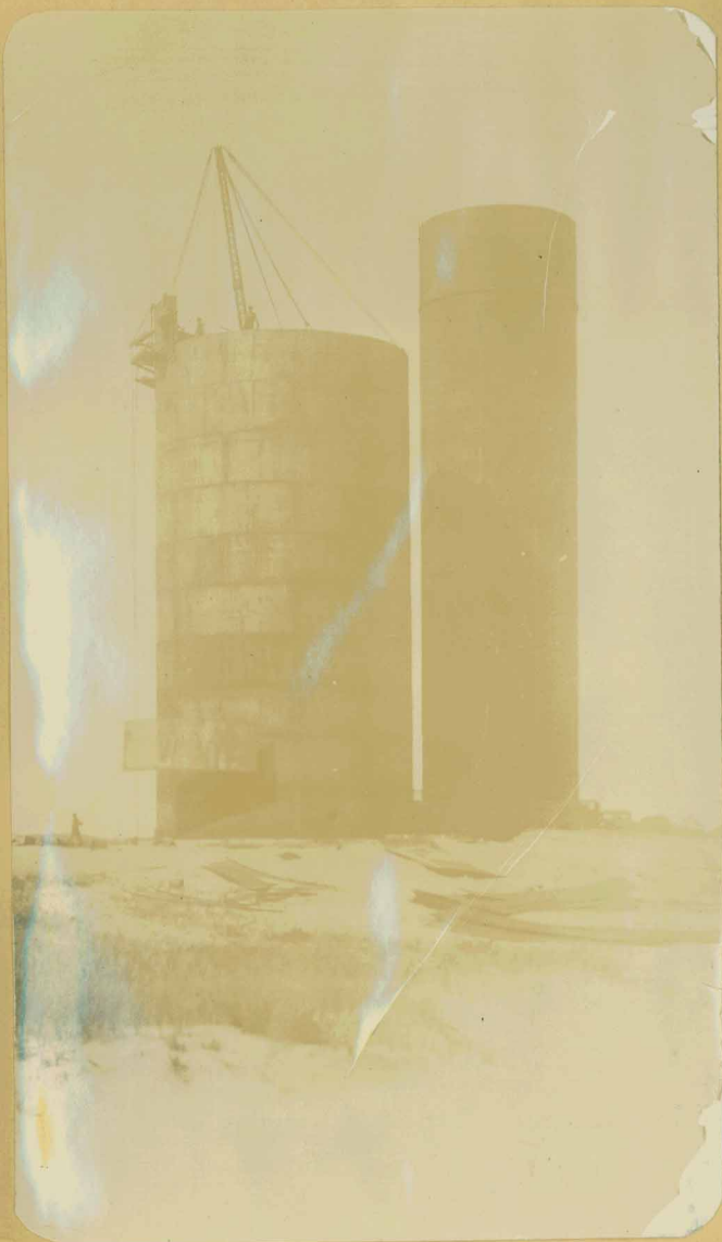
The new standpipe, with the old one beside it. - 1930 -
