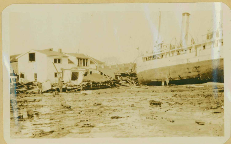
Facing East. Note Pickert's Canning Factory in background (cupolas)
