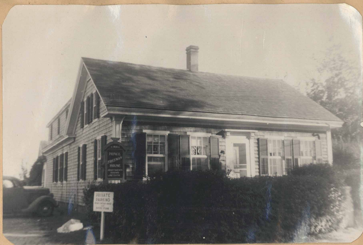
The Prince Freeman House Built 1818 and floated across from Long Pt. Picture taken Sept. 1951
