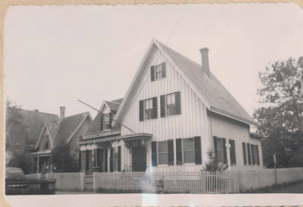
The Houses on Miller Hill facing the wonderful view of the Harbor.
