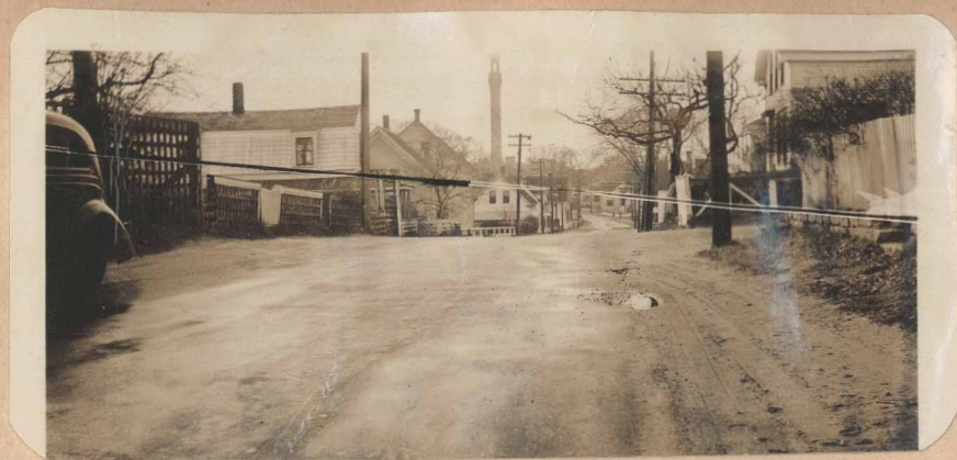
Back on Bradford Street , facing West - 1939 The Monument from Miller Hill.
