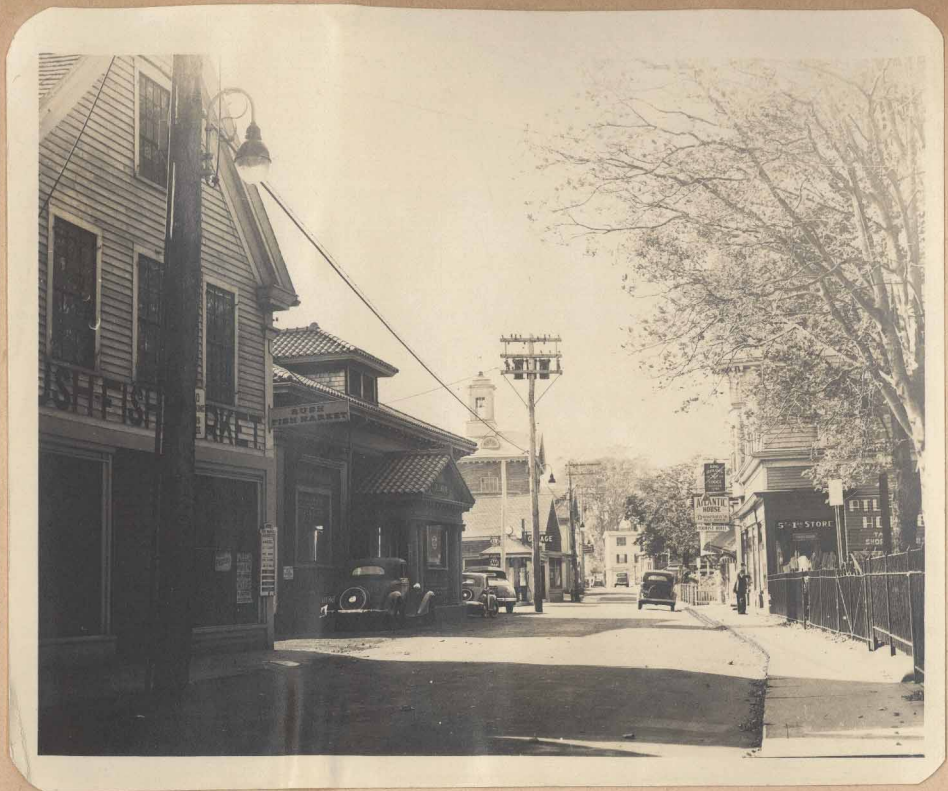
Facing upstreet, west, from the Theatre. Old Storage, left. New Post (Cupola) Note new fence (right) Ben Lancy house (Museum, see pre- ceding pictures)..... John R. Smith - 1940
