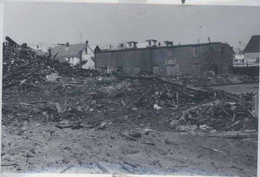
Demolished ATLANTIC COAST FISHERIES - (TUNA FACTORY intact behind Demolition site) MARCH-1975-033-335a-624-068
