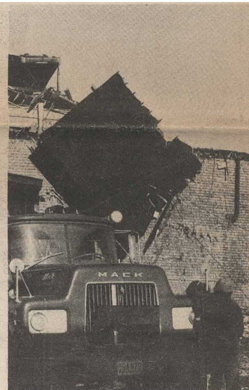
A large section of the roof sails through the air.
