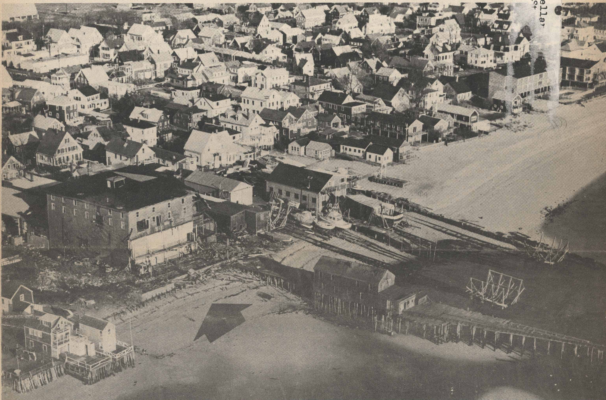
The Coast Guard released its proposal this week for a search-and-rescue station at the Cape Cod Cold Storage plant site in Provincetown. (See story page 6). Arrow points to building with wharf and trap shed bottom right. The plant's razing is a sidewalk superintendent's dream. (See photos page 9.)
