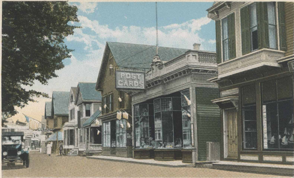
COMMERCIAL STREET OPPOSITE TOWN HALL, PROVINCETOWN, MASS.
